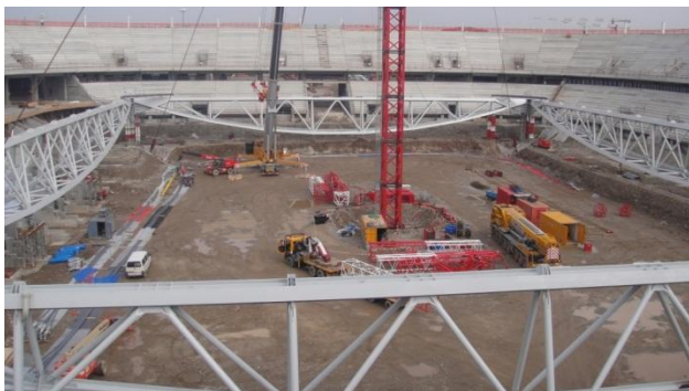
Figure 19: Lifting of the main trusses
