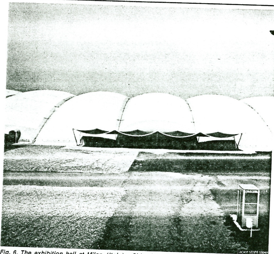
Fig. 6. The exhibition hall at Milan (Italy). Side view of the entrance. Note the parallel cables placed every 15 m.
