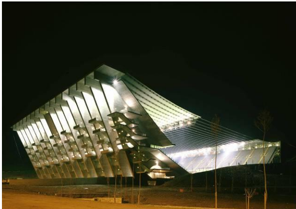
Figure 15. The new suspended cable roof of Braga Stadium (Portugal)
