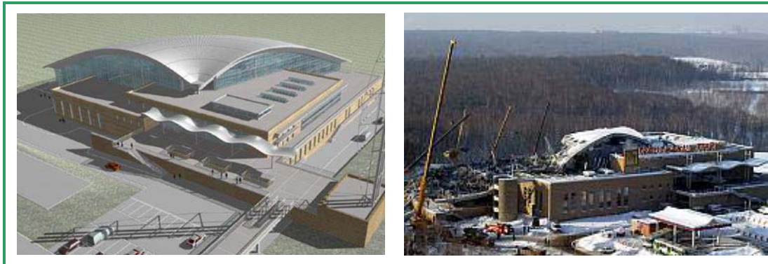
Fig.7 Acquapark and swimming hall Moscow – Roof collapse (2004)
