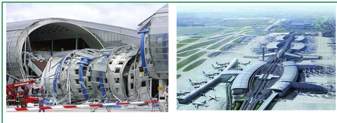
Fig.8 Terminal Roissy Airport Paris – Shell collapse (2004)
