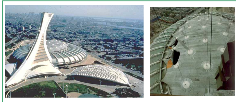
Fig.4 Olympic Stadium Montreal – Roof failure under wind action (1988)
