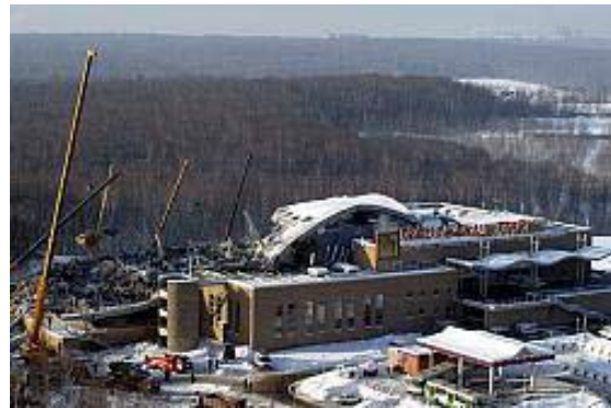
Fig.11 Acquapark and swimming hall Moscow – Roof collapse (2004)
