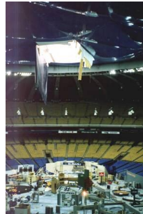
Fig.8 Olympic Stadium Montreal – Partial roof collapse by snow accumulation (1995)
