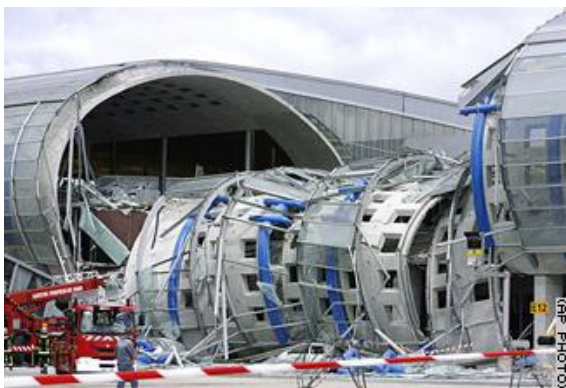
Fig.12 Terminal Roissy Airport Paris – Shell collapse (2004)
