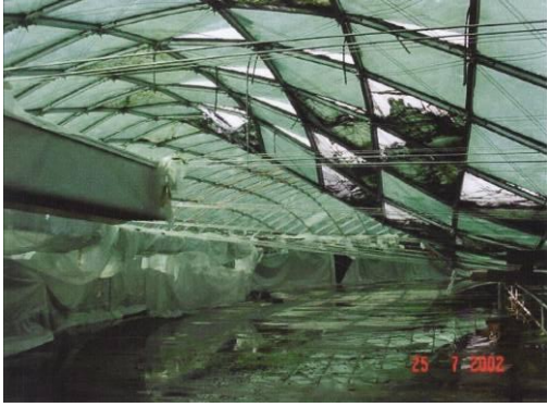
Fig.10 Sport Hall Halstenbeck – Global instability collapse (2002)
