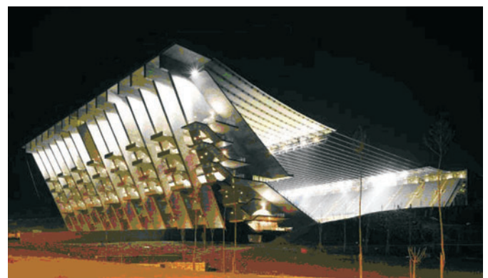
Fig. 30. The new suspended cable roof of Braga Stadium (Portugal)
