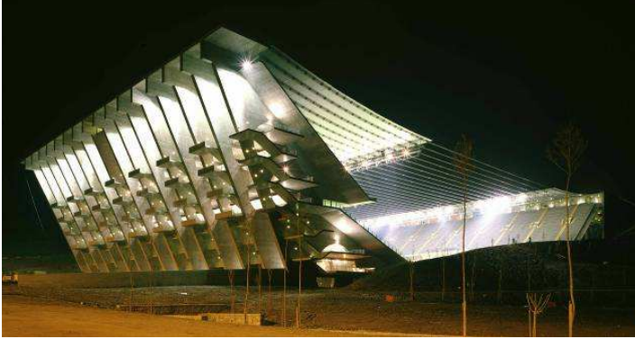
Fig. 34: The new suspended cable roof of Braga Stadium (Portugal)
