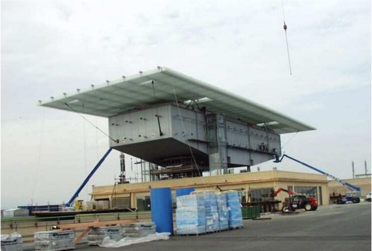
Fig.34. The “Flying Carpet” roof of Lingotto (Turin): example of application of a damping system [132].
