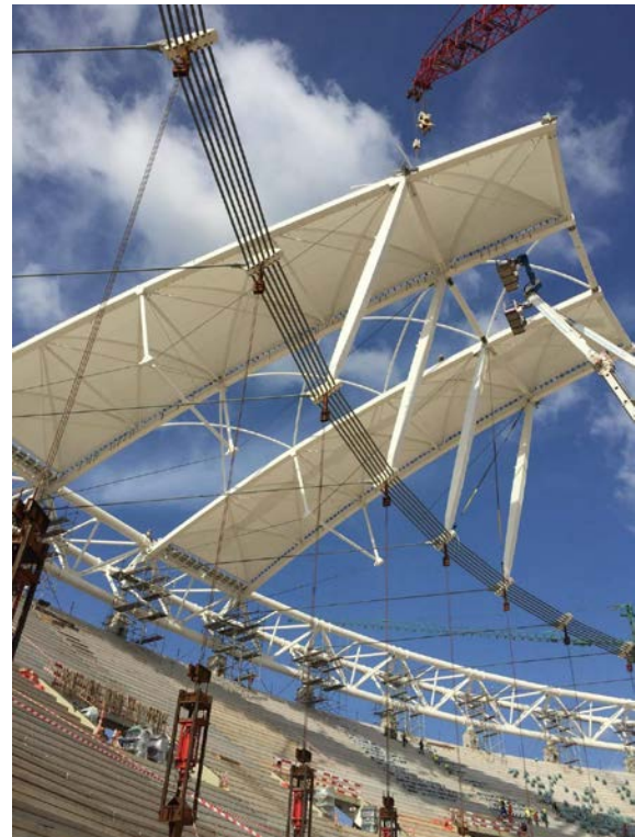
Figure 7-b: Installation of the hybrid radial beams
