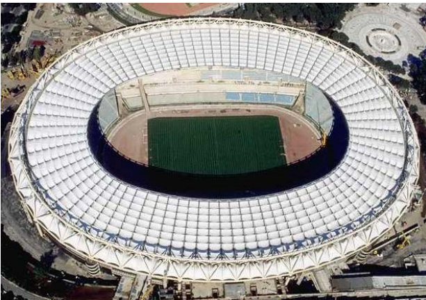
Figure 1-b: Rome Olympic stadium new roof: Prof. Majowiecki solution
