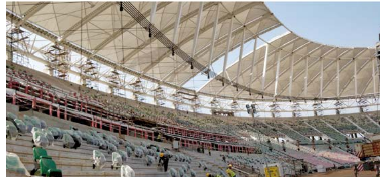
Fig. 18 - Erection sequence: removing of tie down cables
