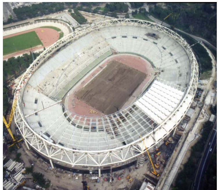
Fig. 7 - Installation of secondary elements and membrane cladding on the cable structure
