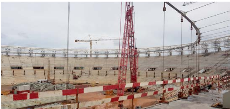
Fig. 17 - Erection sequence: installation of tie down cables
