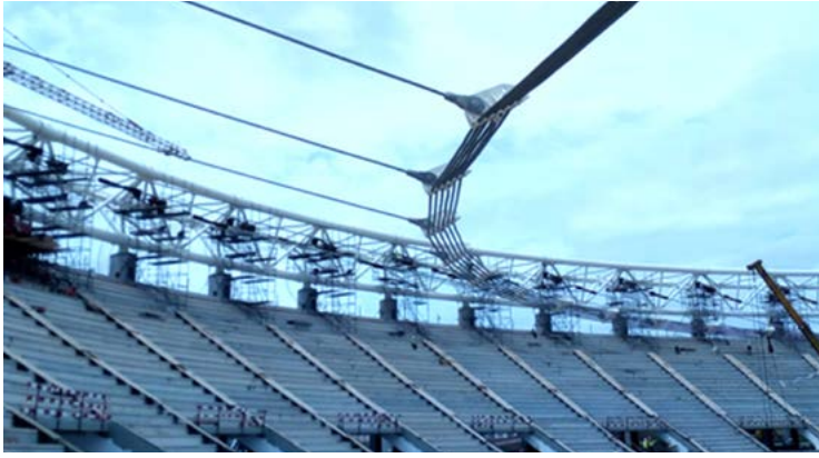
Fig. 16 - tension ring lifted up
