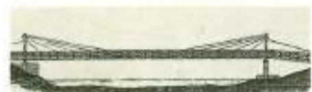
Fig. 1.11 King's Meadows Bridge (Inghilterra 1818).
